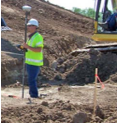
Surveying, Staking, Checking
