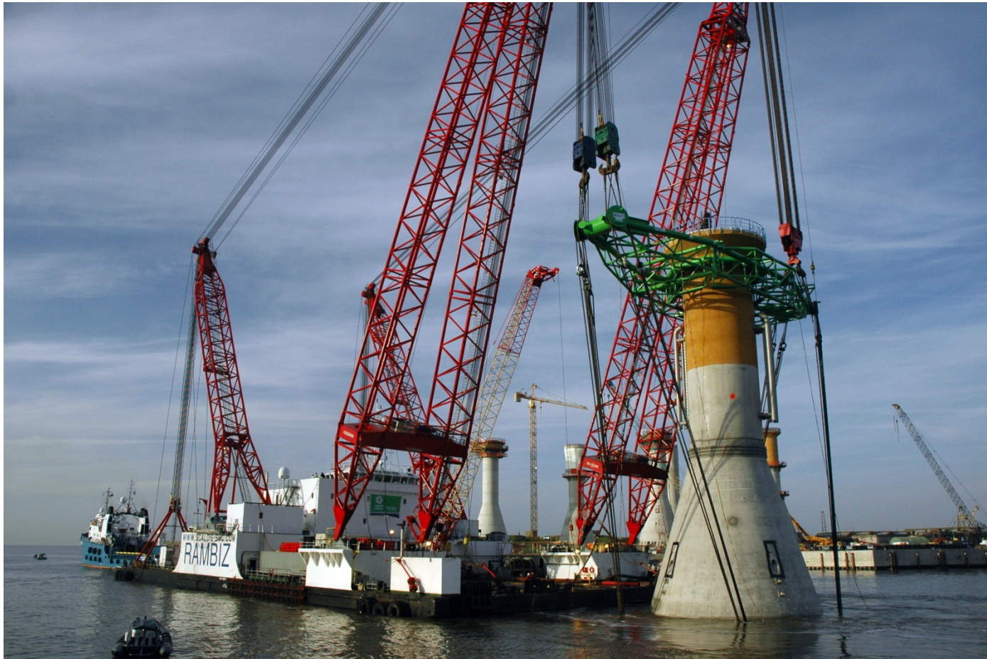
Gravity Based Foundation, C-Power, Thorntonbank
