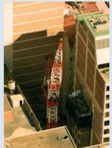
Favelle M230D with 27.4 m short jib and 7.23 m tail radius in the shadow of nearby buildings raising a concrete core in Sydney
