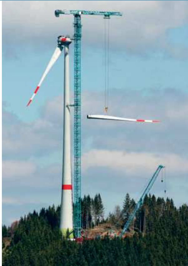
The Liebherr 1000 EC-B 125 Litronic tower crane erecting the Enercon wind turbine
